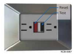
Figure 9-9: Testing GFCI Receptacles
